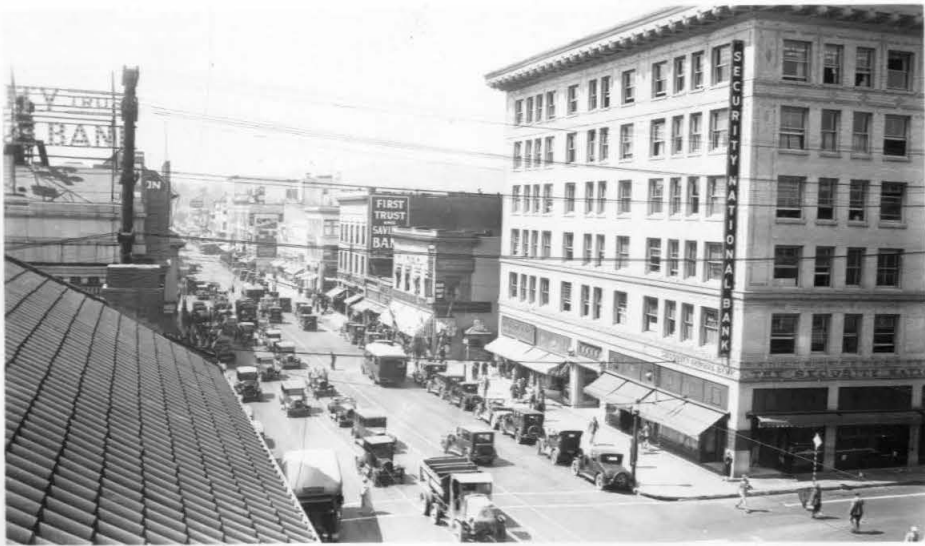
Traffic Delays - Colorado Street
