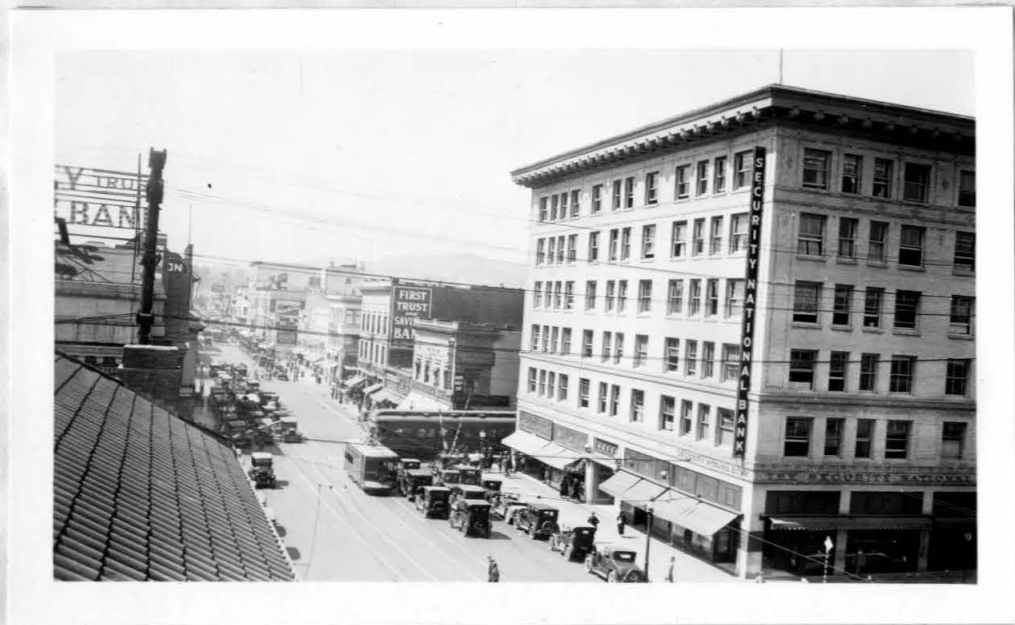
Traffic Delays --- Colorado Street
