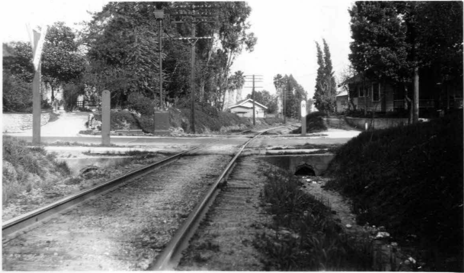
Dangerous Crossing at Wilson Avenue
