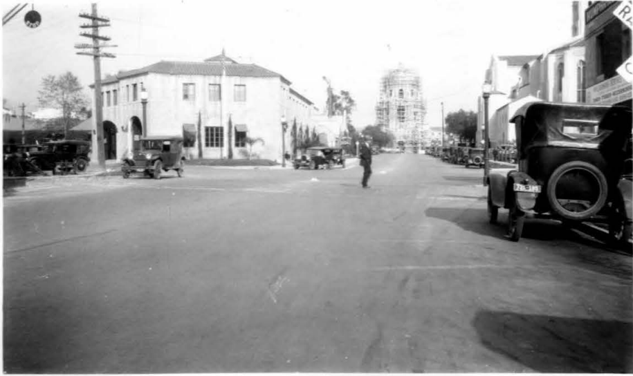
Holly Street Crossing The new City Hall and Civic Center
