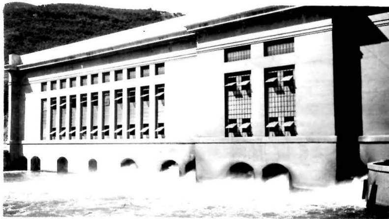
South Front of Power House No.I, San Francisquito Canyon.
