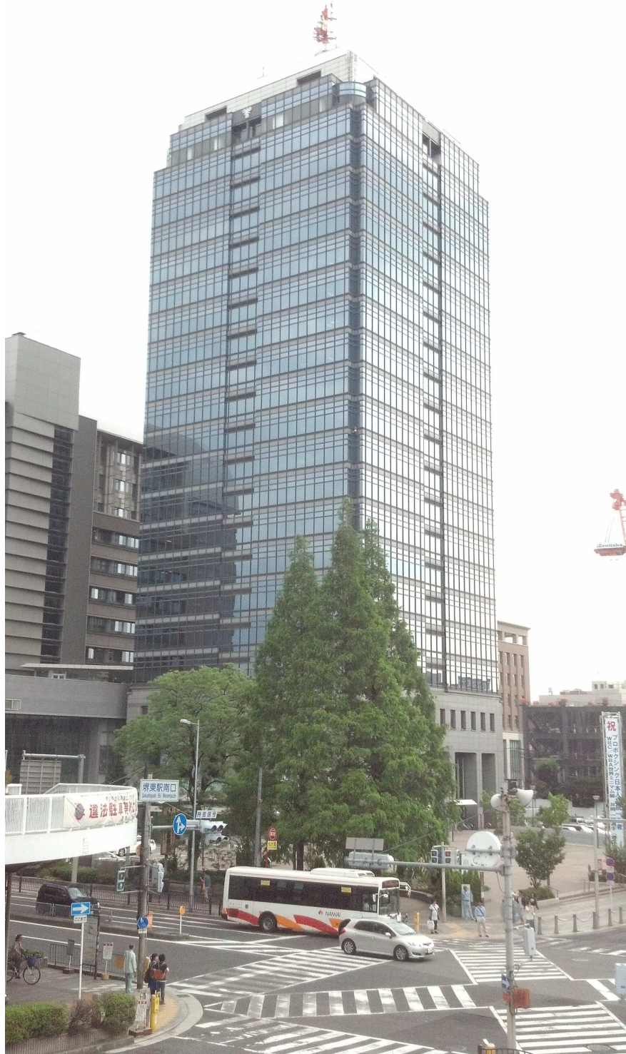
Figure A.4: Osaka High-Rise: Photo of the Building. The building, shown in Figures A.4 and A.5, has 21 stories with two stories for the penthouse, and four stories under the ground level. It is a steel moment-resisting frame above ground and a steel-reinforced concrete frame with shear walls under the ground level.
