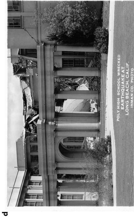
Figure 1.3: 1933 Long Beach Earthquake: Collapse of Unreinforced Masonry Buildings] Postcards documenting the collapse of unreinforced masonry buildings during the 1933 Long beach earthquake, including **a**, a garage at Ocean Blvd, **b**, East Anaheim stores, **c**, a pharmacy, and **d**, the Long Beach Polytechnic High School. Images courtesy of the George W. Housner collection.
