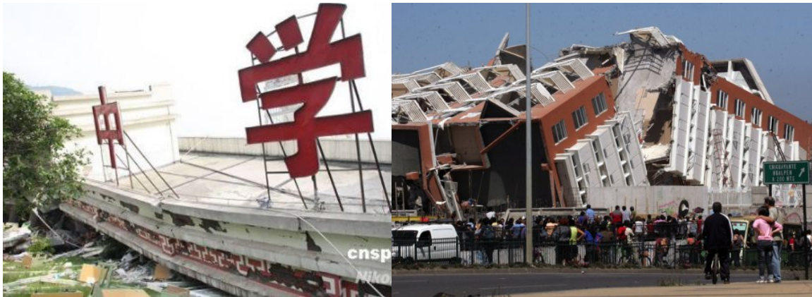
(c) Wenchuan Middle School building collapsed in 2008 Wenchuan earthquake
