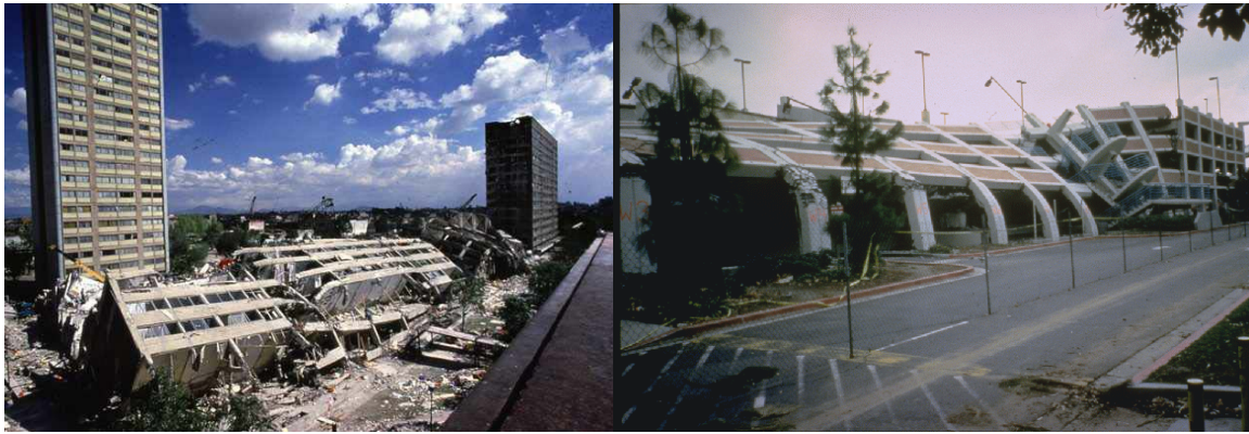
(a) The Nuevo Leon apartment building collapsed in 1985 Michoacán earthquake
