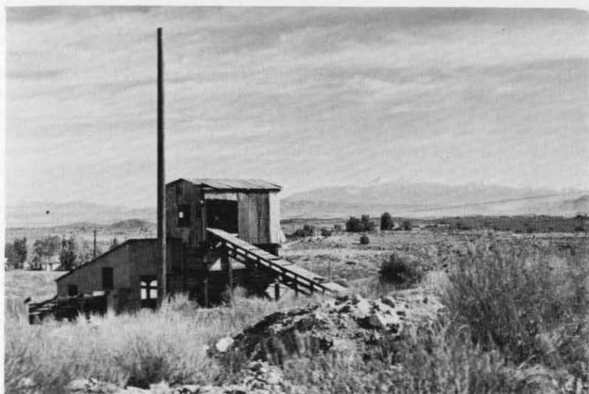
FIGURE 3. View eastward of Good Hope mill building, long inactive, with mine dump in foreground, Perris surface is in near background, Mount San Jacinto on right skyline. Photo by Mort D. Turner, 1954.
