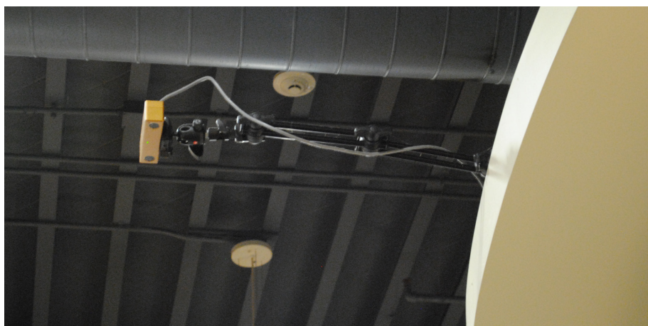
Figure D.4: Camera networking and power. Gray cord is firewire line carrying both.
