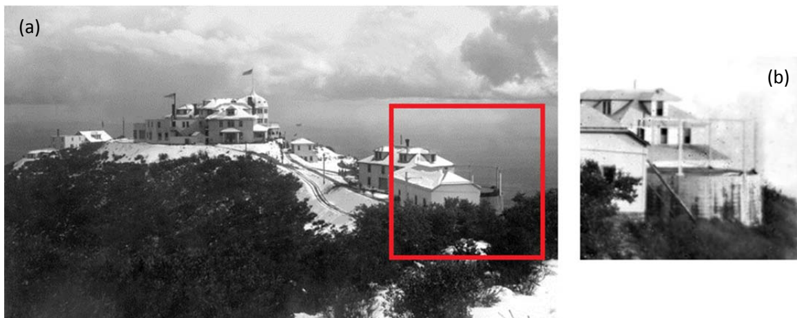
Figure 1.2. (a) The Echo Mountain House and Mt. Lowe Railway shown in 1893. An inflatable hydrogen storage container is shown in the red box. (b) A close-up view shows the framework used to support the gas reservoir which would expand upon filling.
