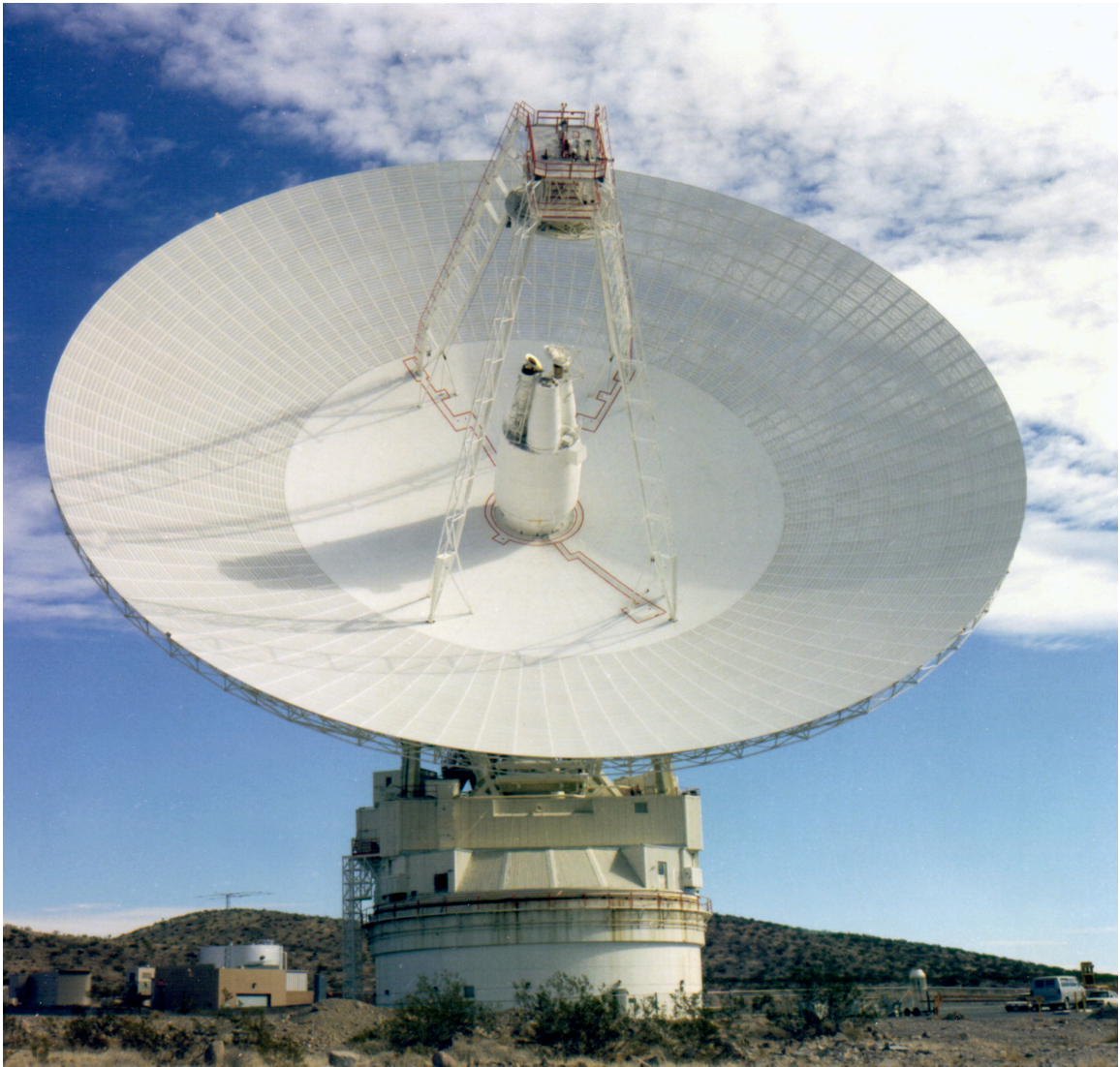
Figure 3.1: (b), Goldstone Deep Space Network, Mojave Desert, California, 70-m steerable antenna. The transmitter and receivers are mounted in separate feed horns at the Cassegrainian focus.
