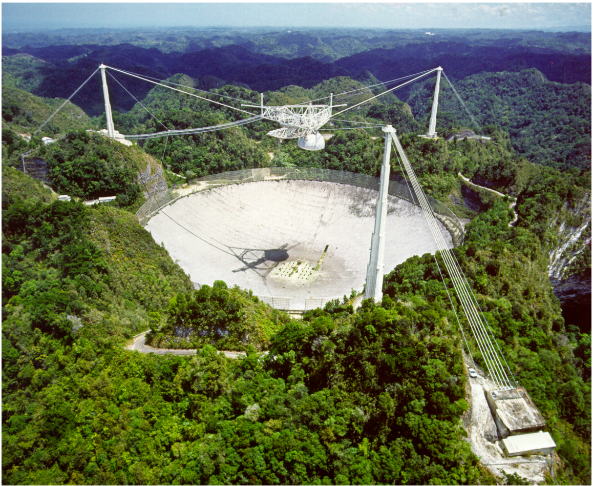
Figure 3.1. (a) Arecibo Observatory, Puerto Rico. The antenna is a 305-m fixed spherical dish. The transmitter and receivers are mounted inside the Gregorian dome on the platform and moved to permit pointing within roughly 20^\circ of zenith.
