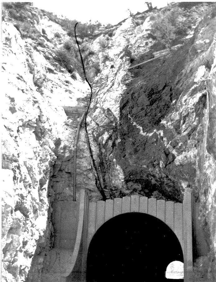
Fig. 69 Goat fault at the west portal of the new road tunnel in Soledad Canyon.
