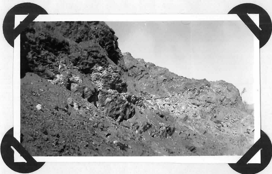
View showing the trace of the San Francisquito Fault crossing the St. Francis Dam Site.
