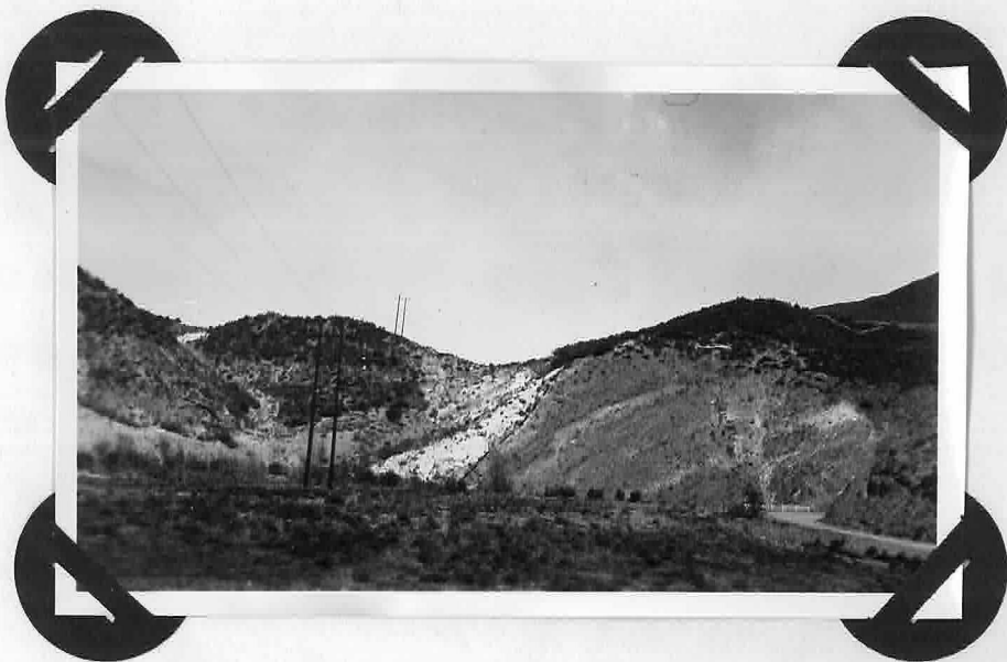
Looking north at a section of the San Francisquito Fault, showing the Le Brun formation thrust over the Pelona schist. View taken adjacent to Power House No. 2, below the St. Francis Dam Site.
