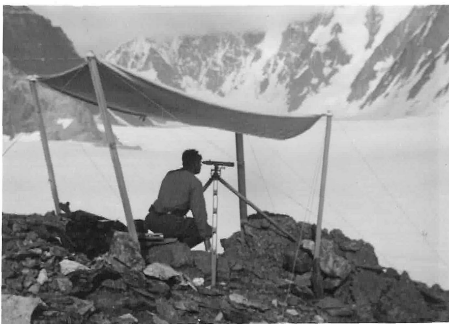
Fig. 13. Observation of glacier movement through level.
