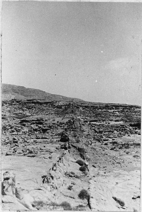
Fig. 13 Igneous dike cutting almost at right angles through tilted Eocene sandstones and shales. The comparatively even surface is the scoured and dissected platform of the fifth island stage as revealed on the south side of the island. Note the absence of in-fill.
