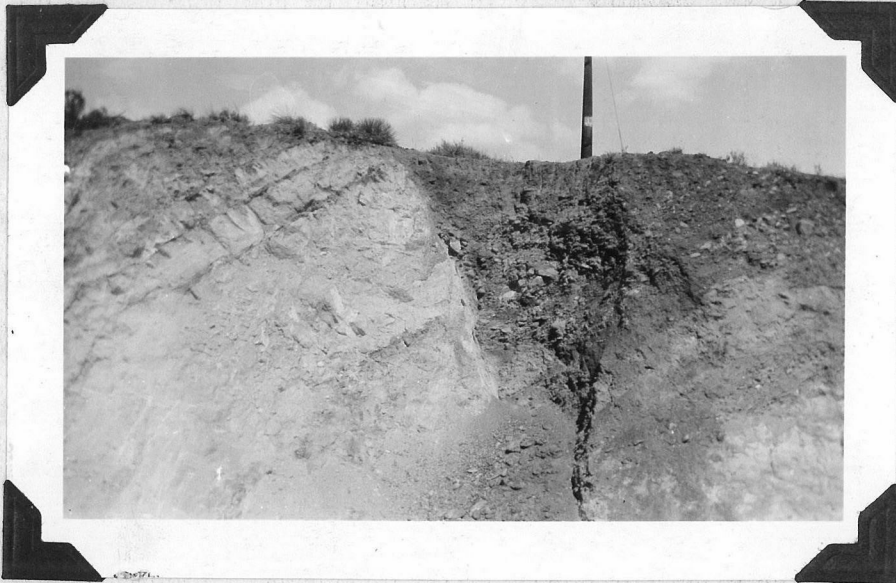
Figure 28 - One of the Faults of the San Andreas Zone, Near Palmdale, Cal. (On State Highway)
