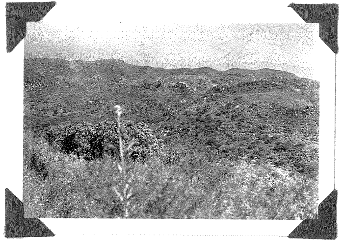
Figure 2. View of west dike, west of northern part of Laguna Canyon. Showing abnormal induration of sediments near intrusive contact. (Page 38)
