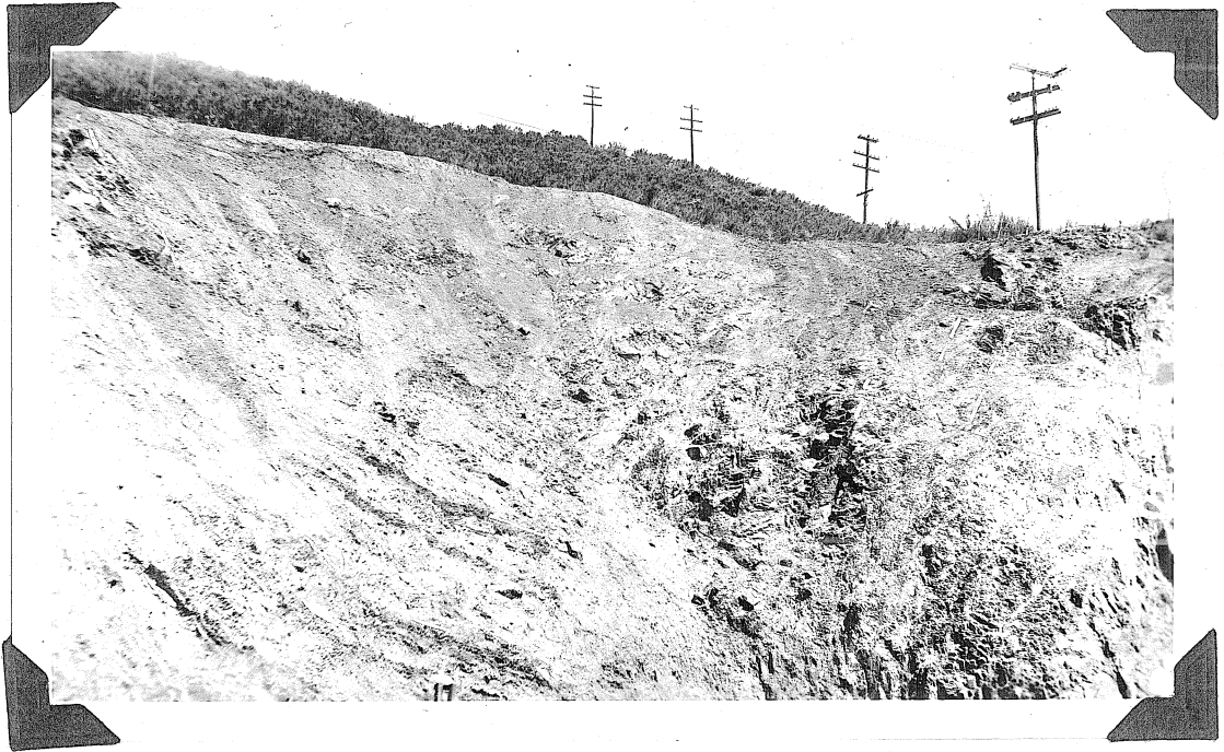
West Clearwater Canyon. Slumping of the shales within the Martinez(?) formation.
