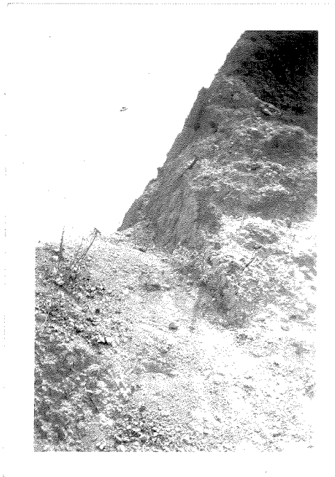
Fig. 22 Slickensided surface of fault E On highway 1500' NE of Workman Hill Point
