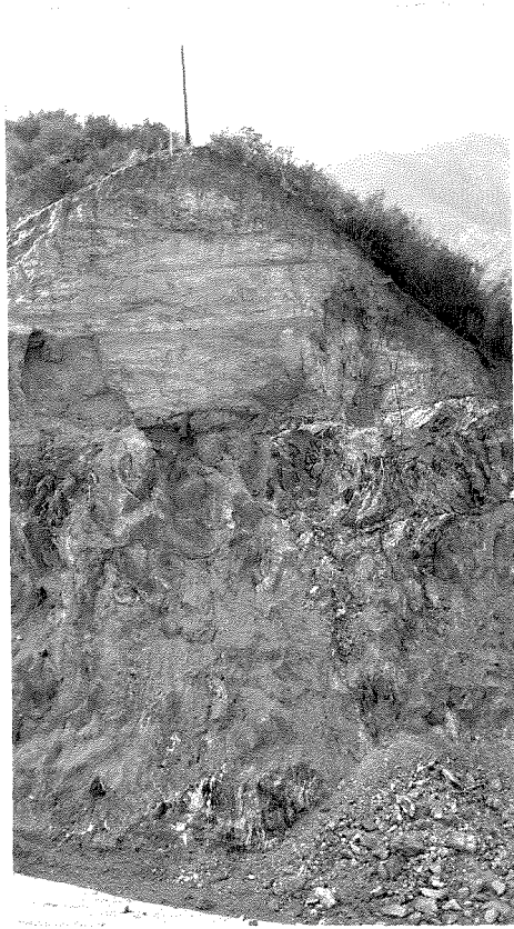
Exposure of Little Tujunga Fault in road cut in Little Tujunga Canyon
