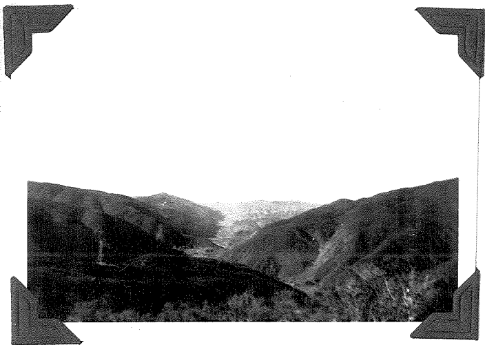
Fig. 37. San Francisquito Fault, San Francisquito Canyon.
