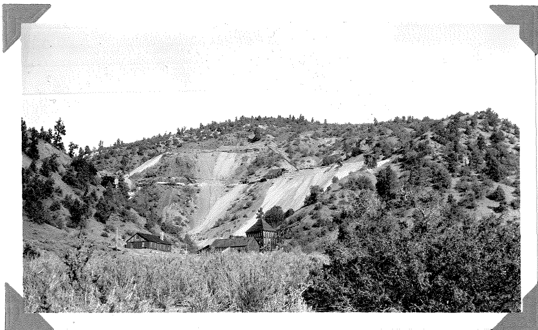
Fig. 23. Frazier borax mine (abandoned) on north side of Lockwood Valley. Colemanite was mined from lenses of limestone and colemanite interbedded with basalt flows.
