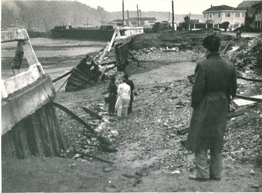
FIGURE 1.14 - FAILURE OF SHEET-PILE SEA WALL AT PUERTO MONTT - FROM (11)
