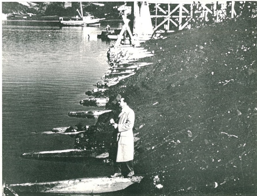
FIGURE 1.13 - PUERTO MONTT, GRAVITY WALL FAILURE - FROM (11)
