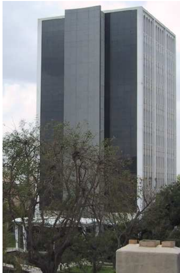
Figure B.1: Robert A. Millikan Memorial Library: View from the northeast. The dark colored walls in the foreground comprise the East shear wall.
