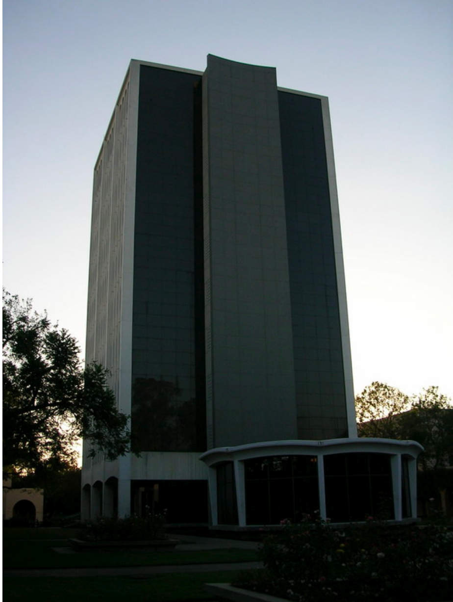
Figure A.2: Caltech Millikan Library. View from the South-East. The dark grey walls in the foreground are structural shear walls, and the white panels on the south (left) side of the building are non-structural marble cladding.
