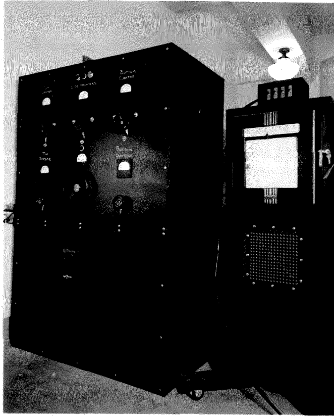
Figure 9. Heater Controls and Temperature Recorder
