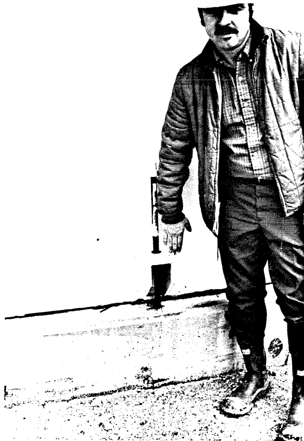
Figure 1.6 Uplift at the Tank Bottom (San Fernando, 1971, Ref. [3])
