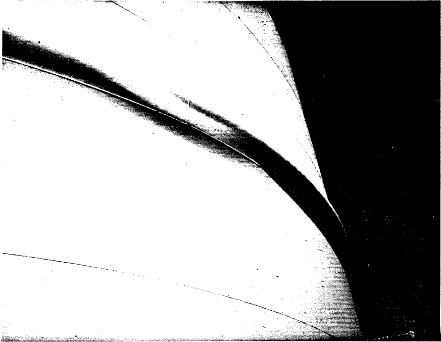
Figure 1.3 Buckling at a Middle Section of a Tank
