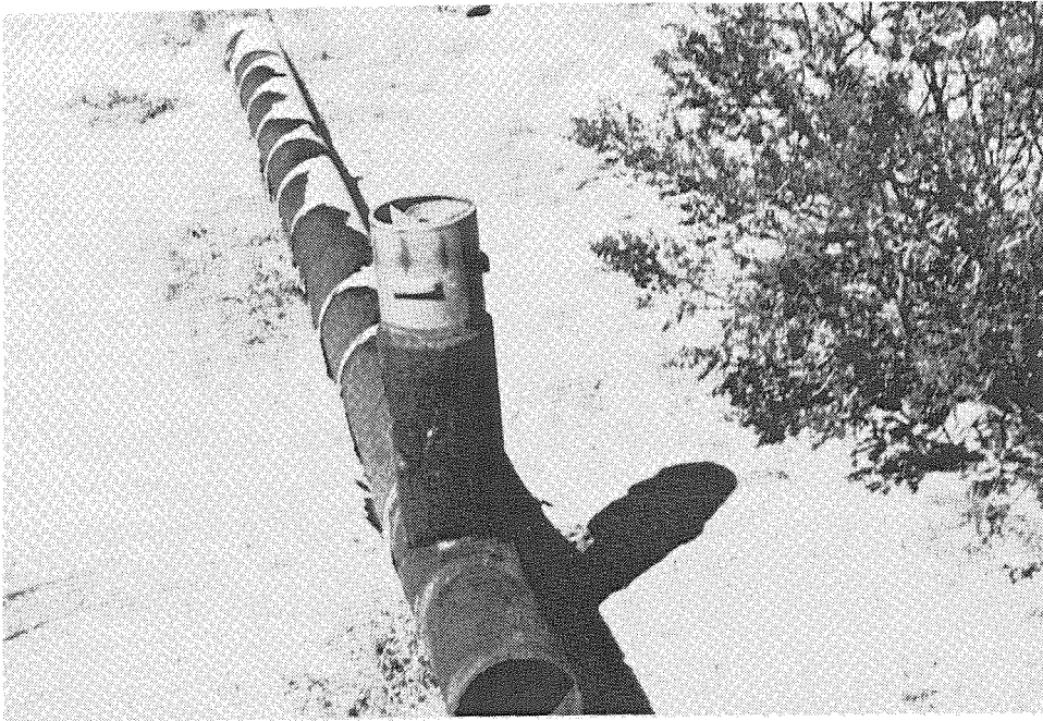
Figure 4: Photograph of old abandoned flood irrigation system in primary study area. When this system was being used, there would be a cap at the top of the vertical pipe forming an alfalfa valve which could be opened and closed to regulate the water flow.
