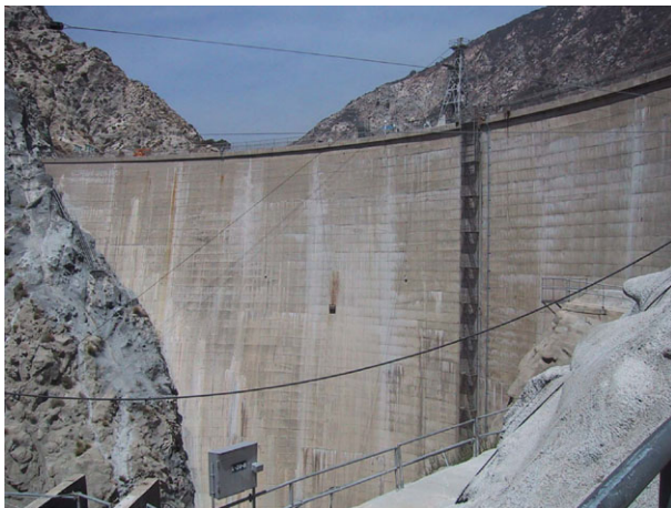
(a) View of right abutment
