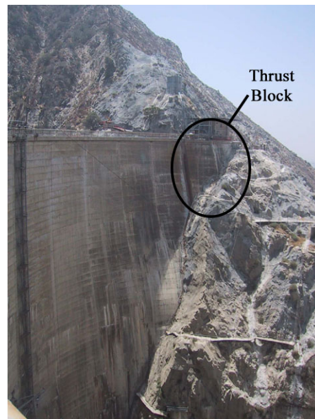
(b) View of left abutment
