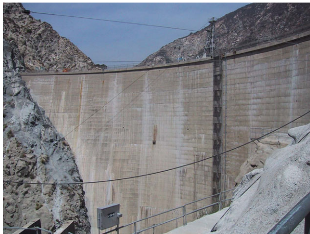
(a) View of right abutment
