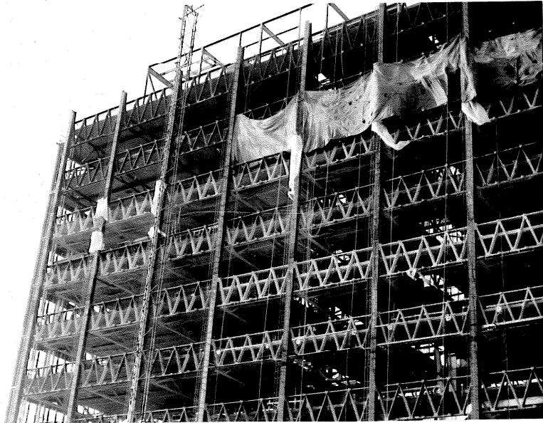
Fig. A-6 EXTERIOR VIEW, LOOKING NORTHWEST.
