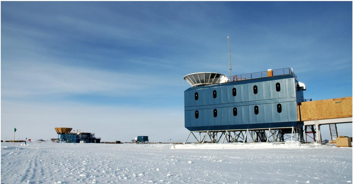
Figure 4.1: The Dark Sector Laboratory at the South Pole Station, where BICEP is deployed. Further back to the left, the MAPO building houses the QUAD experiment on the DASI mount.
