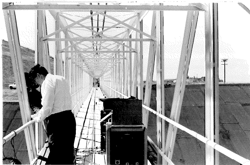
VIEW OF BRIDGE, LOOKING TOWARDS DAM
