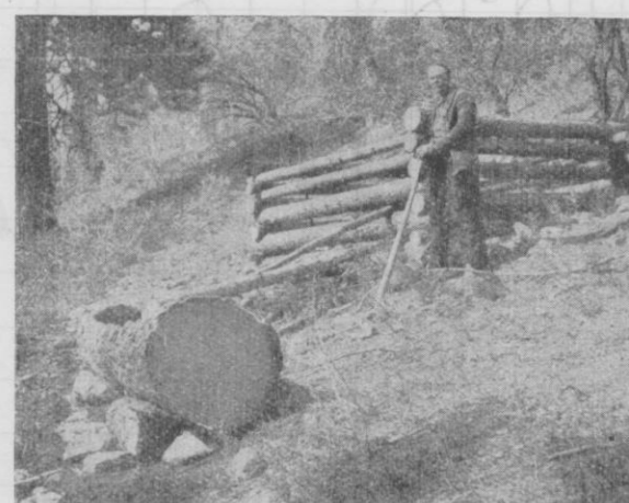
Spring Fenced and Water Piped into Trough for Stock
