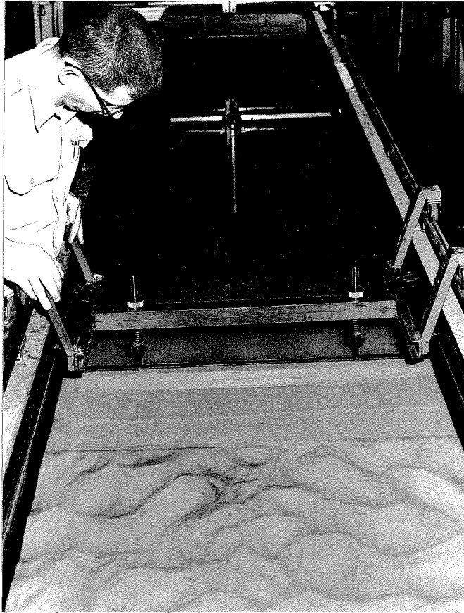
Fig. 3-12. Bed-leveler for 60-foot flume.
