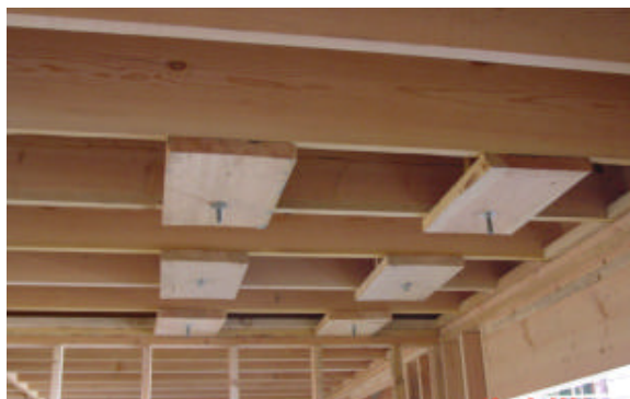
Figure 5.14: Shaker Setup (view of second floor ceiling)
