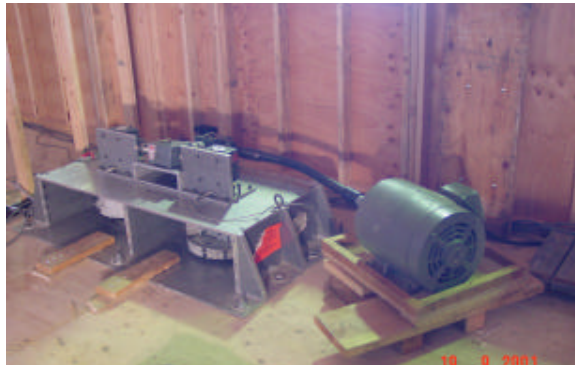
Figure 5.13: Shaker Setup (third floor)
