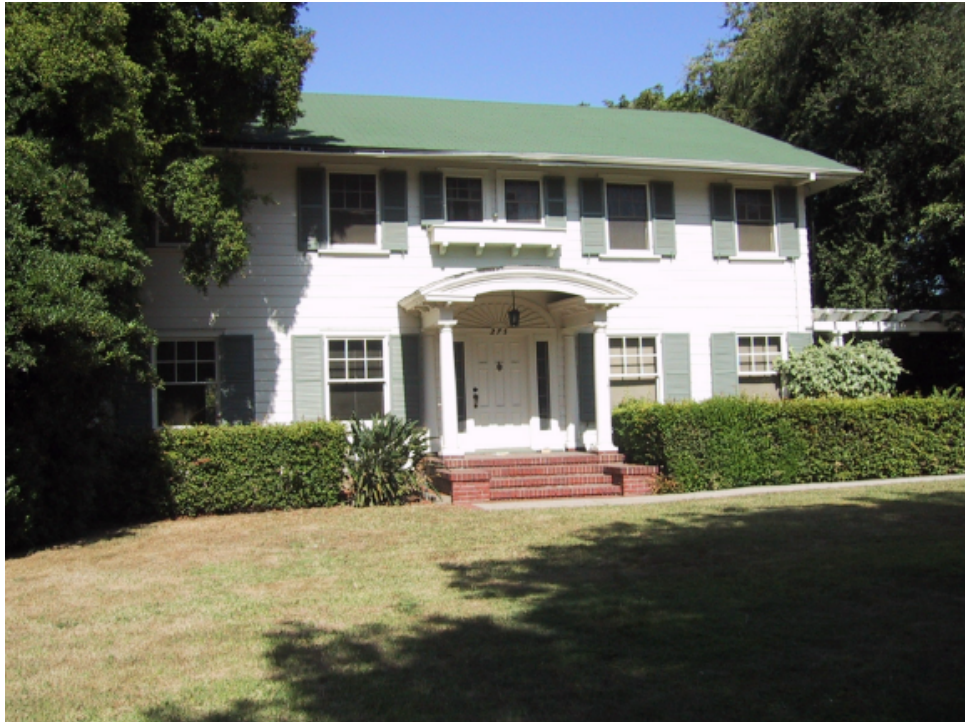
Figure 4.32: 2-Story House on S. Hill Ave., Pasadena
