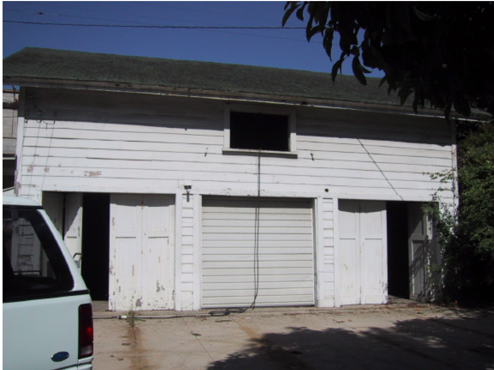
Figure 4.26: 2-Story Garage on S. Hill Ave., Pasadena
