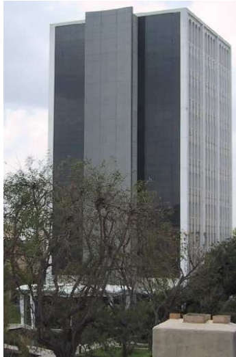
Figure A:1. Robert A. Millikan Memorial Library: View from the Northeast. The two dark colored walls in the foreground comprise the East shear wall.
