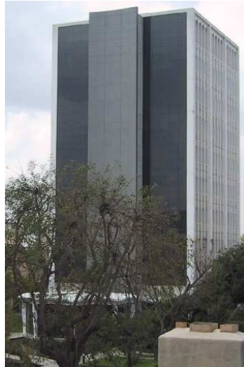
Figure A:1. Robert A. Millikan Memorial Library: View from the Northeast. The two dark colored walls in the foreground comprise the East shear wall.
