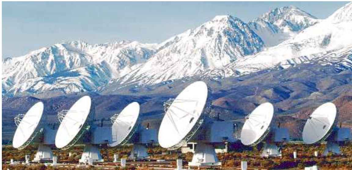
Figure 2.10 A photograph of the Owens Valley Millimeter Array (OVRO). OVRO consists of six 10.4 m telescopes, located on the East side of the high Sierra Nevada.
