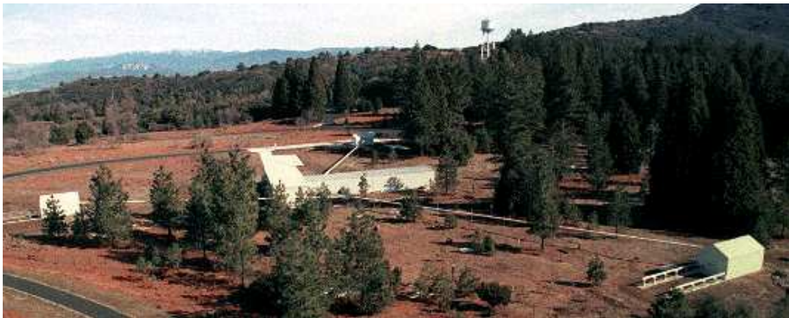
Figure 2.7 A photograph of the Palomar Testbed Interferometer (PTI), courtesy of NASA/JPL-Caltech. The three siderostats reside in small white huts. The North siderostat is in the top middle part of the image, West is on the left, and South is in the lower right corner. Vacuum pipes transport light from the siderostats to a central beam-combining building, which contains the delay lines, beam combiner, and detector.
