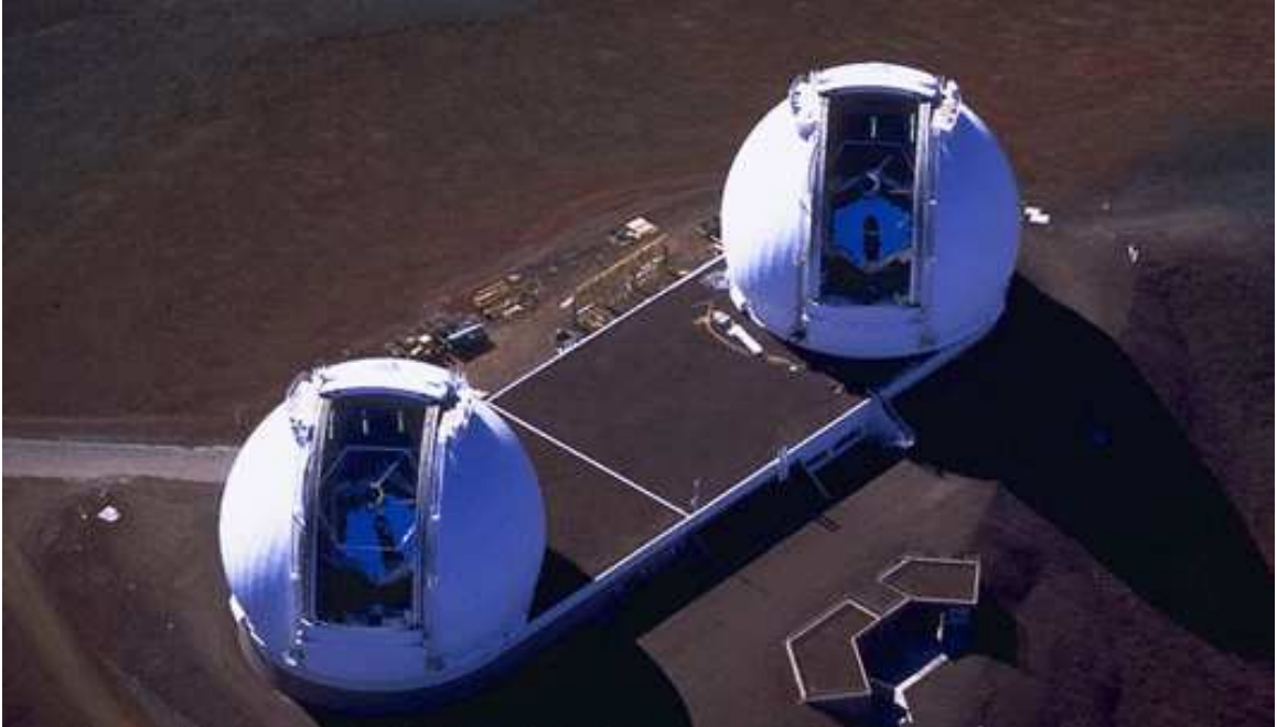
Figure 2.9 A photograph of the Keck Interferometer (KI), courtesy of NASA/JPL-Caltech. KI currently consists of the two 10 m Keck apertures, separated by an 85 m baseline. The basement of the building connecting the two telescopes contains the beam transport system, delay lines, beam combiner, and detector.
