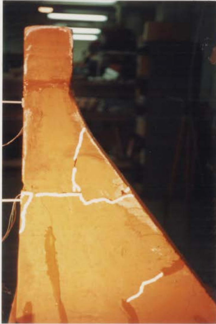
Figure 4.11: (b) Opposite side of monolithic model after initial cracking earthquake test.
