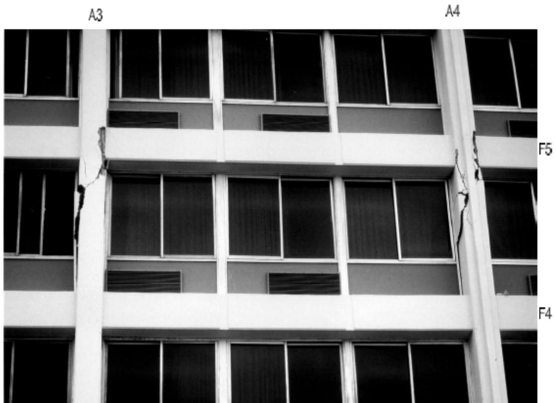
Figure 6.27: Photograph of shear cracks occurring in the south frame of the structure during the Northridge earthquake. Taken from Trifunac et al. (1999).
