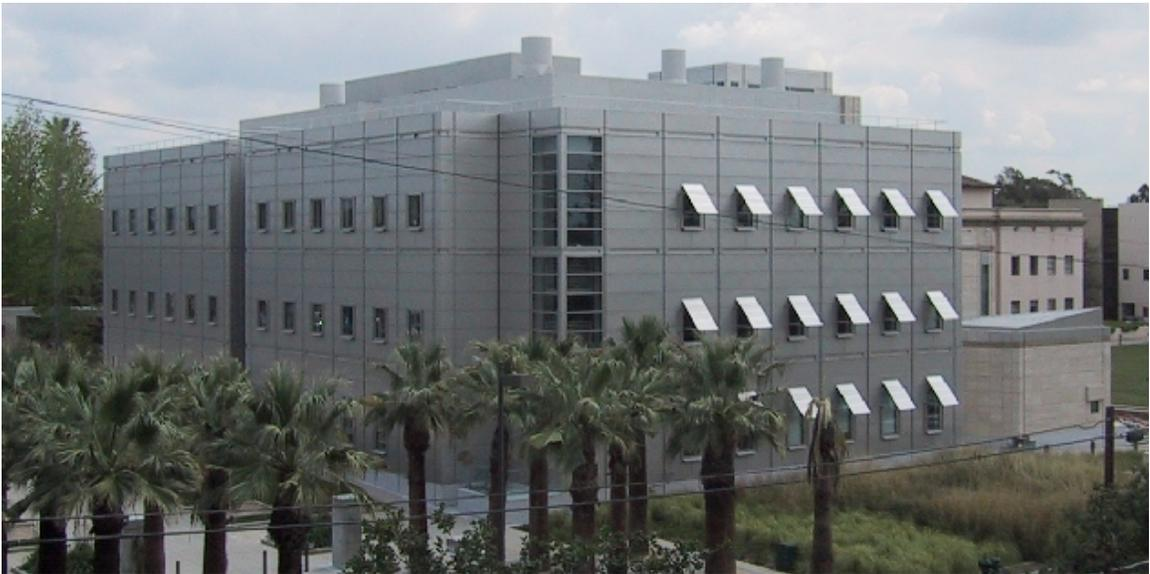
Figure 6.8: Broad Center - View from North-West. Structural core of the unbonded-brace frame is located below the parapet wall visible on the roof (Figure 6.9 contains a plan view).
