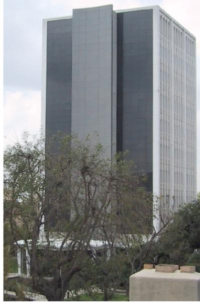
Figure 6.1: Millikan Library - View from North-East. The two dark coloured walls in the foreground comprise the 30.5cm thick east shear wall, which is somewhat narrower on the ground floor, due to walkway openings. The wall panels and concrete moment frame are visible on the north face
