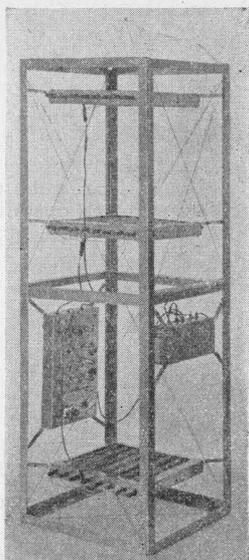
FIG. 3. The components were shock mounted in an aluminum framework. The weight of the whole assembly including 1800 cm<sup>2</sup> of counter area was 8 kg.
