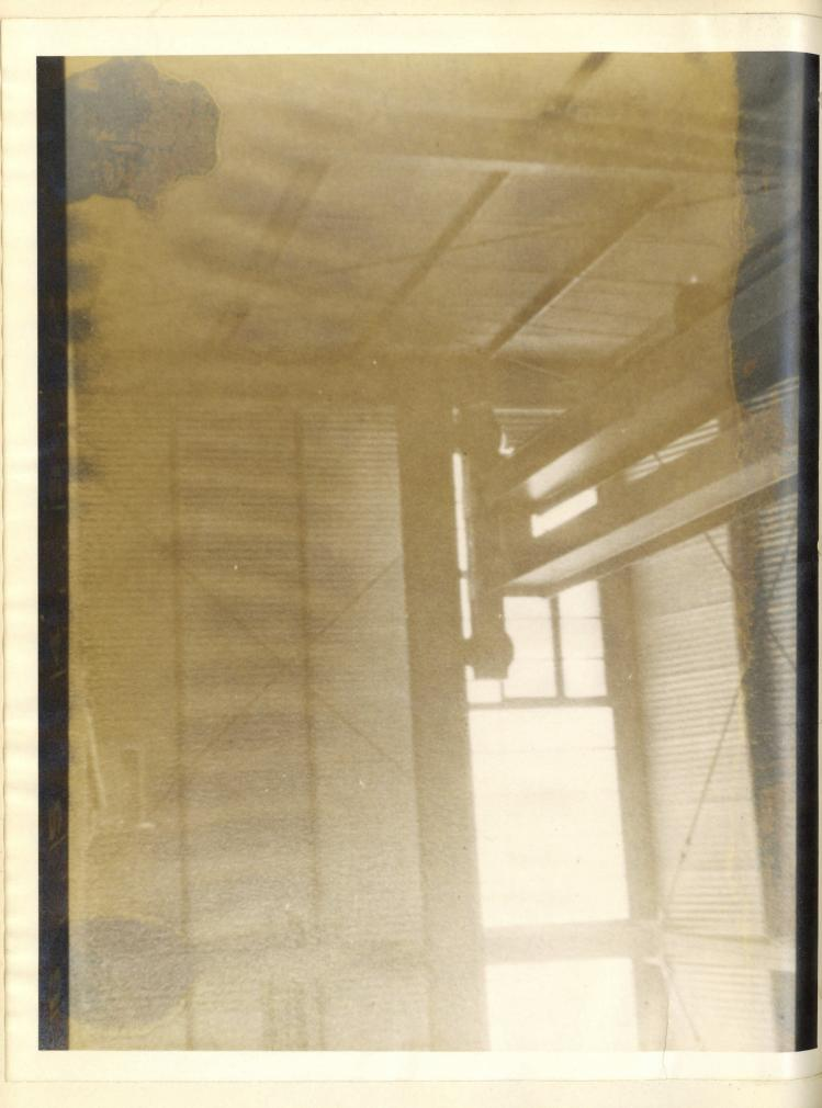
The south building appears to have deflected very little, less than an inch for even the weak "D" wall. Although this wall deflected most, the resultant diagonalrod stress is quite low because of the inadequacy of the rod bracing system. The considerable unbraced length of the columns along this wall accounts for the greater part of the deflection.
