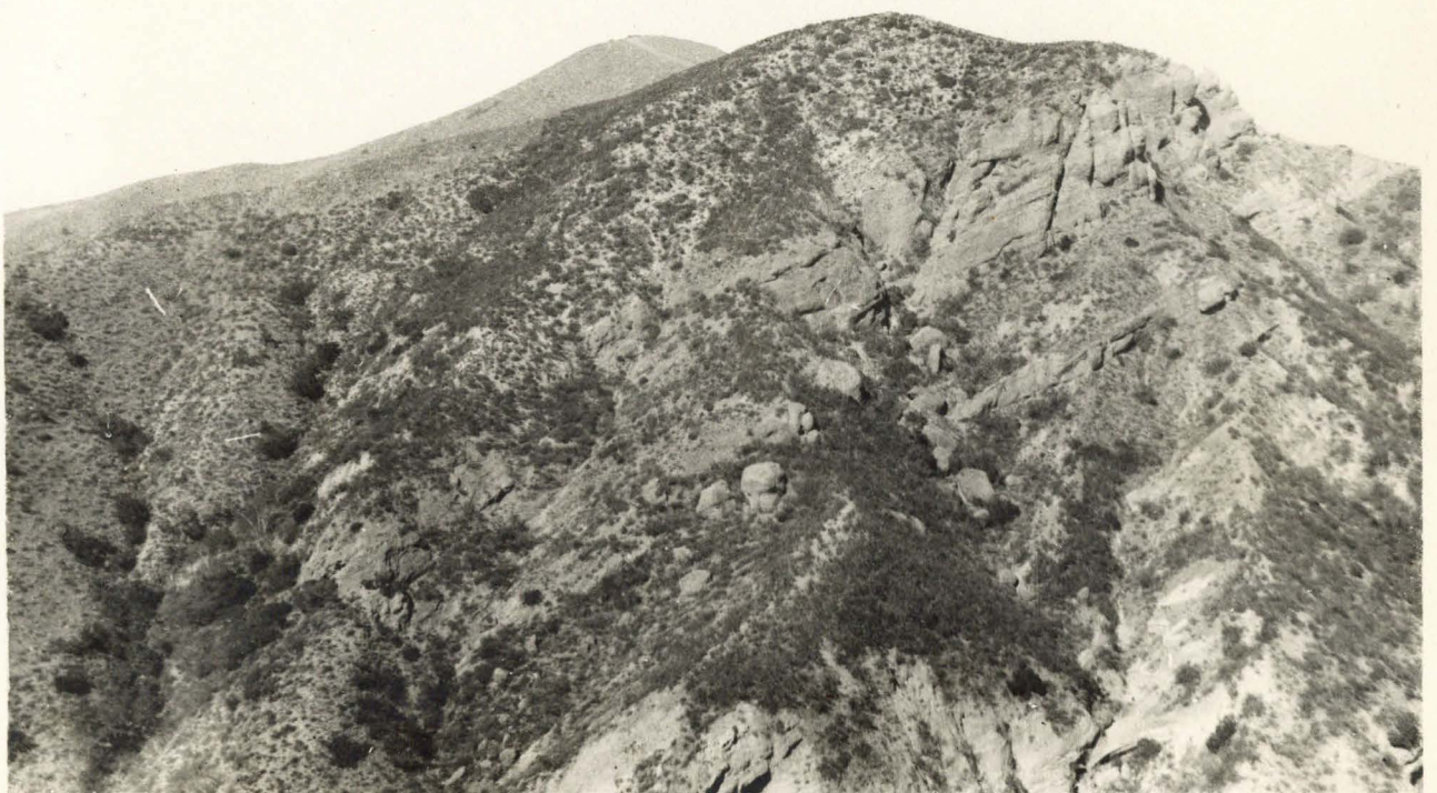
Fig 2. View Looking North Across Harding Canyon in the Vicinity of the Dam.
