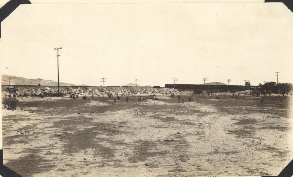
Santa Fe Railroad Bridge at Barstow.
