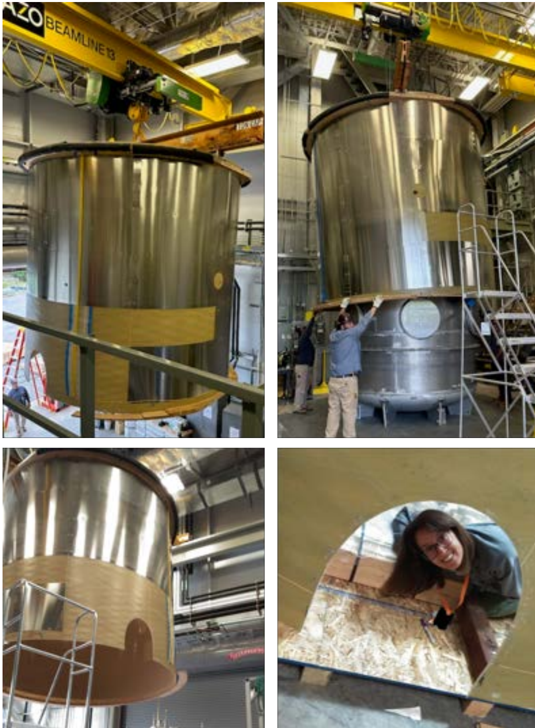
Figure 4.34: Photographs of the mu-metal Shield Installation. Top left, the shield is lifted with a spreader bar. Top right, the shield is lowered around the cryomagnet. Bottom left, the shield is rotated so the IMV services pass through the mouse hole. Bottom right, postdoctoral mouse peeks through the hole for scale.
