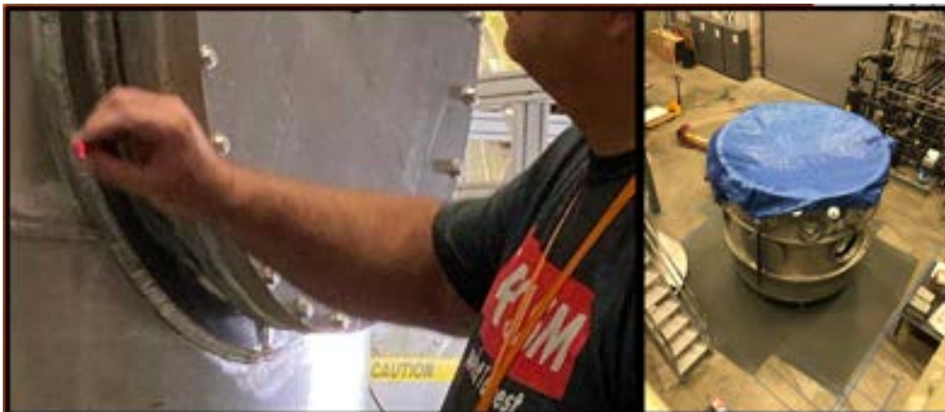
Figure 4.24: Photographs of the OVC placement. Left, the survey and alignment team affixing their laser alignment system to the outside of the OVC. Right, the completed placement of the OVC on the steel plates in the experimental hall.
