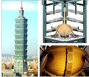
(a) Tuned Mass Damper (TMD): secondary mass moving out of phase with primary structure [13]. Ex: vibration mitigation: Taipei 101, Taipei.
