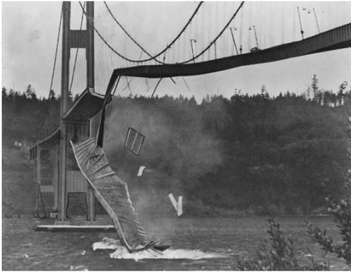
(a) Tacoma Narrows Bridge: wind-induced self oscillation amplified until supporting cables failed, resulting in bridge collapse [1–3].
