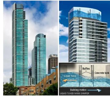
(b) Tuned Liquid Damper (TLD): secondary mass moving out of phase with primary structure [14]. Ex: vibration mitigation: One Rincon Hill, San Francisco.
