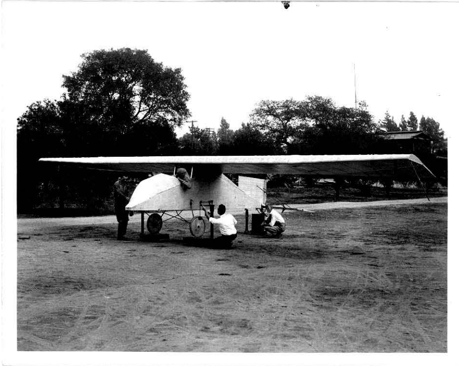
Photo. 28. Locating Center of Gravity. (see Page 20)
