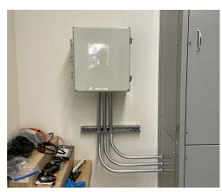
(a) Meter enclosure (right) mounted on the wall and connected via electrical conduits to the main switchboard (left)
