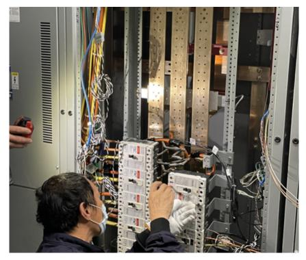
Figure 6.8: Installation of voltage taps via a 20A breaker in the main busbars of Annenberg Center main switchboard MSA.
