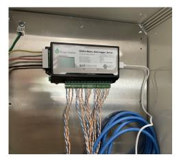
(b) Inside the eGauge meter enclosure. Power/voltage connections are on the left side of the device and CT sensor connections are on the underside. The enclosure chassis is grounded to the switchboard ground bar.
