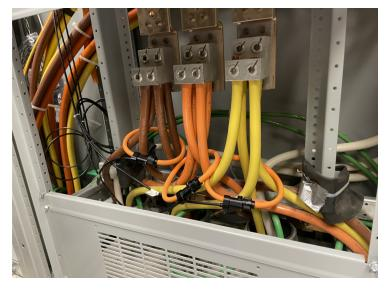
Figure 6.7: 1600A Rogowksi coil CTs (orange loops) on the main lines feeding the busbars of MSB in Annenberg.
