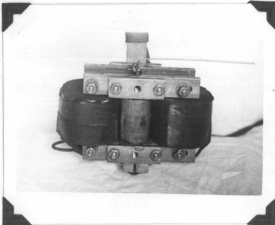
Armature And Field Coils Of Electromagnetic Drive
