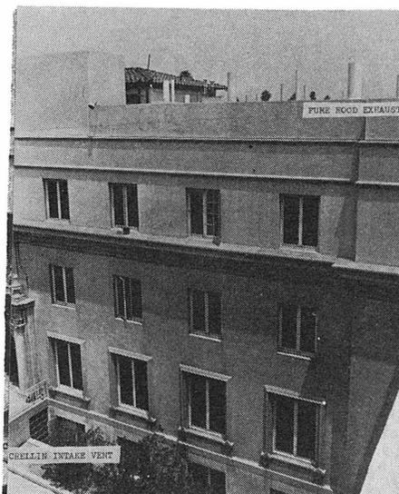
Figure 9. West side of Crellin, showing the fume hood outlet from Room 357 and the ground-level ventilation intake
